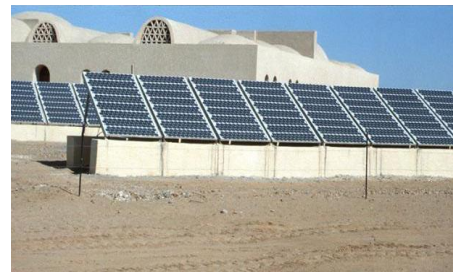
Fig. 3. Solar energy, El-Sadat City, Egypt
